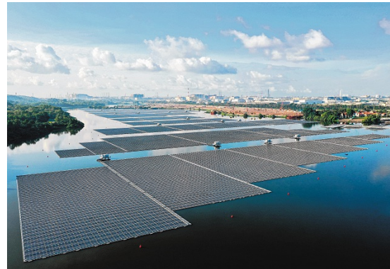
The Sembcorp Tengoh Floating Solar Farm. If the proposed hybrid system is found feasible, the parties involved plan to design and deploy a pilot system with at least 100MW of renewable energy capacity – enough to power 3,000 four-room Housing Board flats a day. This can be scaled up over time. ST FILE PHOTO
